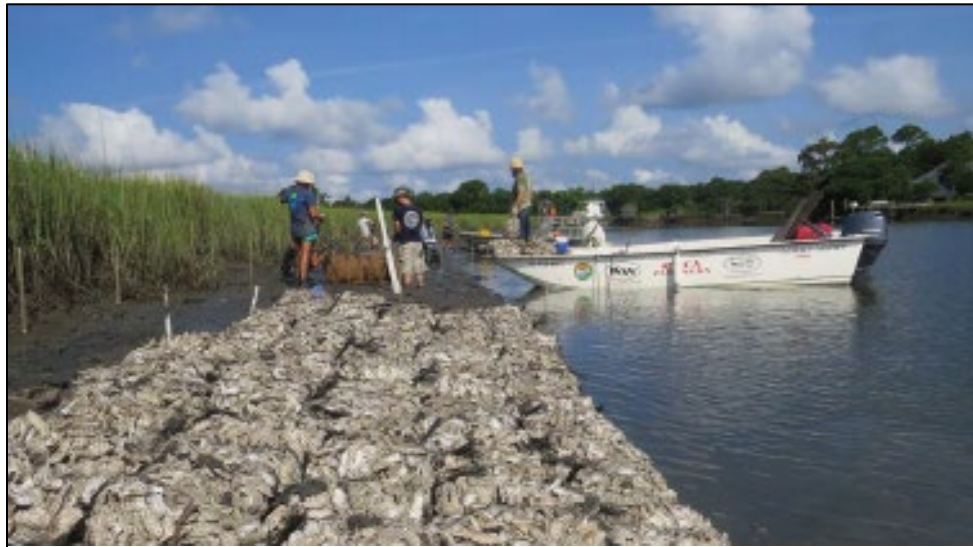
Figure 4. Typical bagged-shell oyster reef sill found in South Carolina. Source: SCDNR
